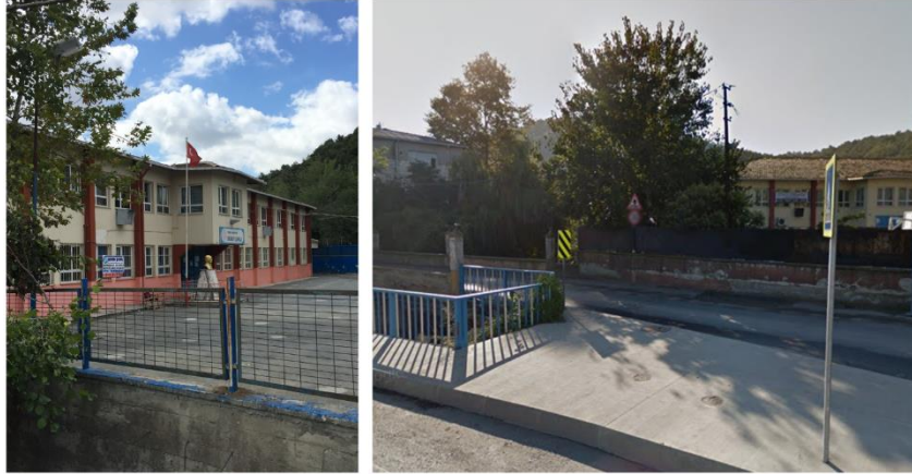
Figure 1-4 Photos of Boğazköy Primary School
