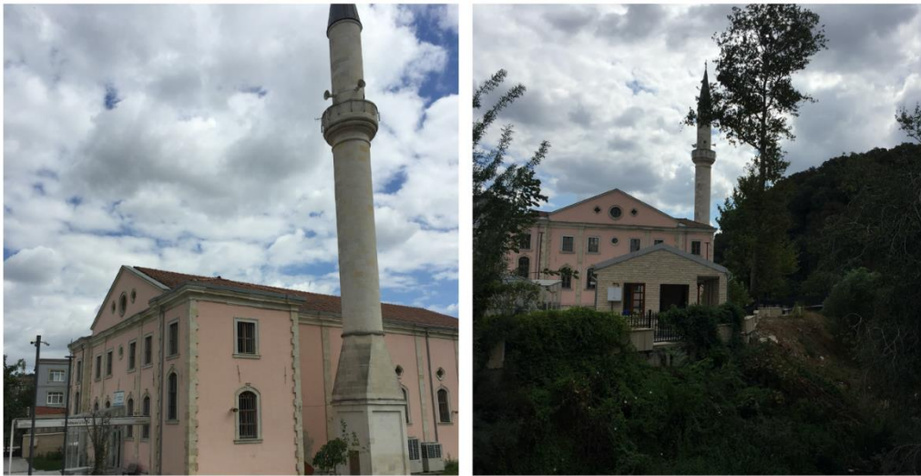
Figure 1-3 Photos of Boğazköy Mosque
