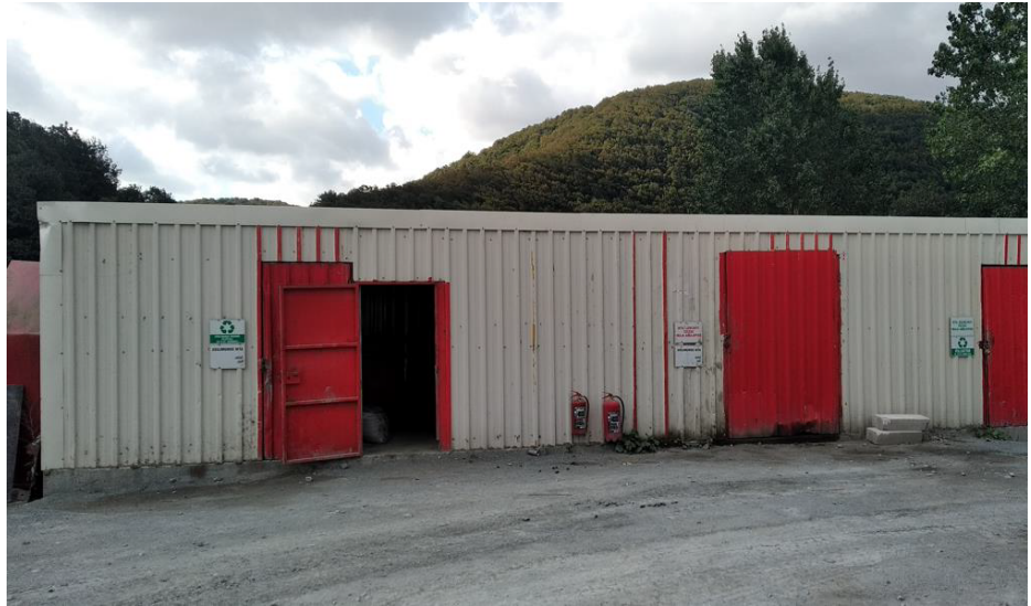
Temporary hazardous waste area
