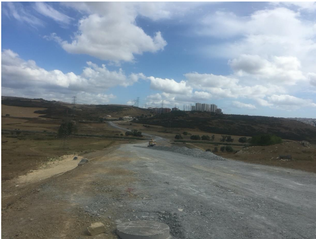
Figure 7-10 Photos of Başakşehir Stray Animal Hospital and Kayabaşı Kiptaş Residence Site
