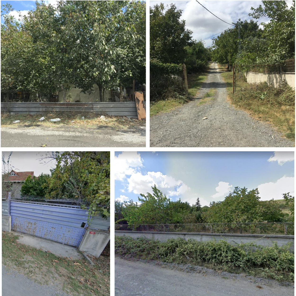
Figure 7-2 Photo's form Muratdere Street Settlements
